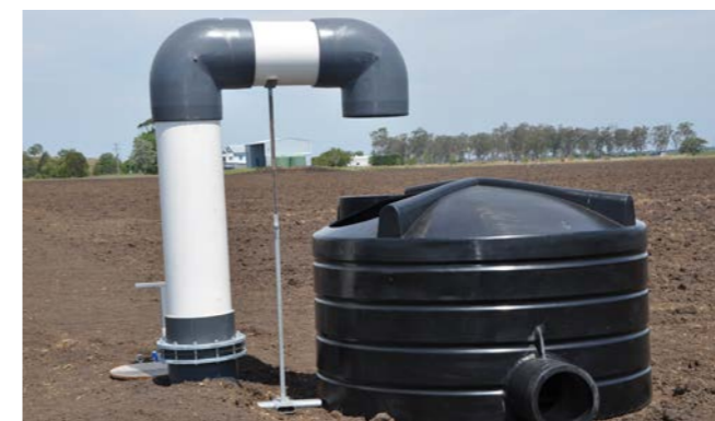
Figure 4.10 – Farm-level irrigation infrastructure supporting controlled water distribution across tea tree plantations. Distributed storage tanks and regulated outlets enable targeted irrigation while avoiding field-wide flooding.
