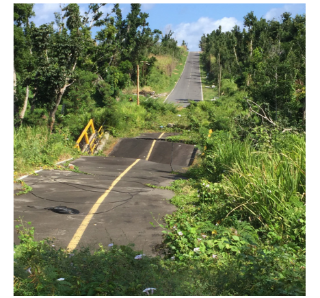
1. A SECTION OF THE MAIN WEST COAST ROAD
